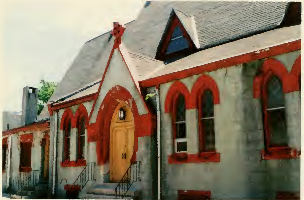
North Elevation of Church Building (L)
